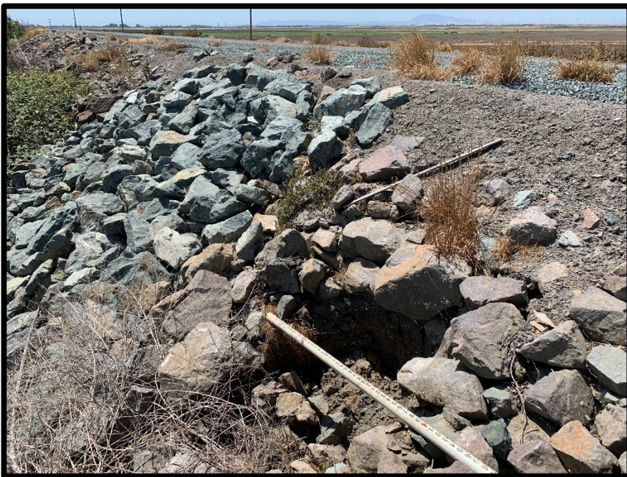
Sink hole on upper slope (Station 219+85).
