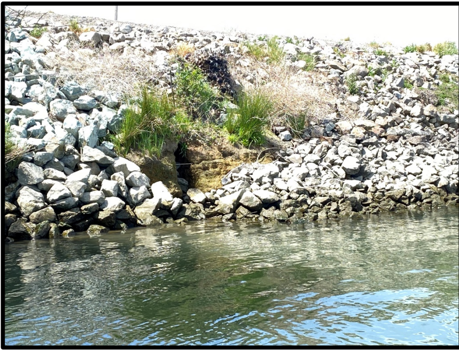
Sinkholes on upper slope and void on lower third of waterside slope (Station 219+85).
