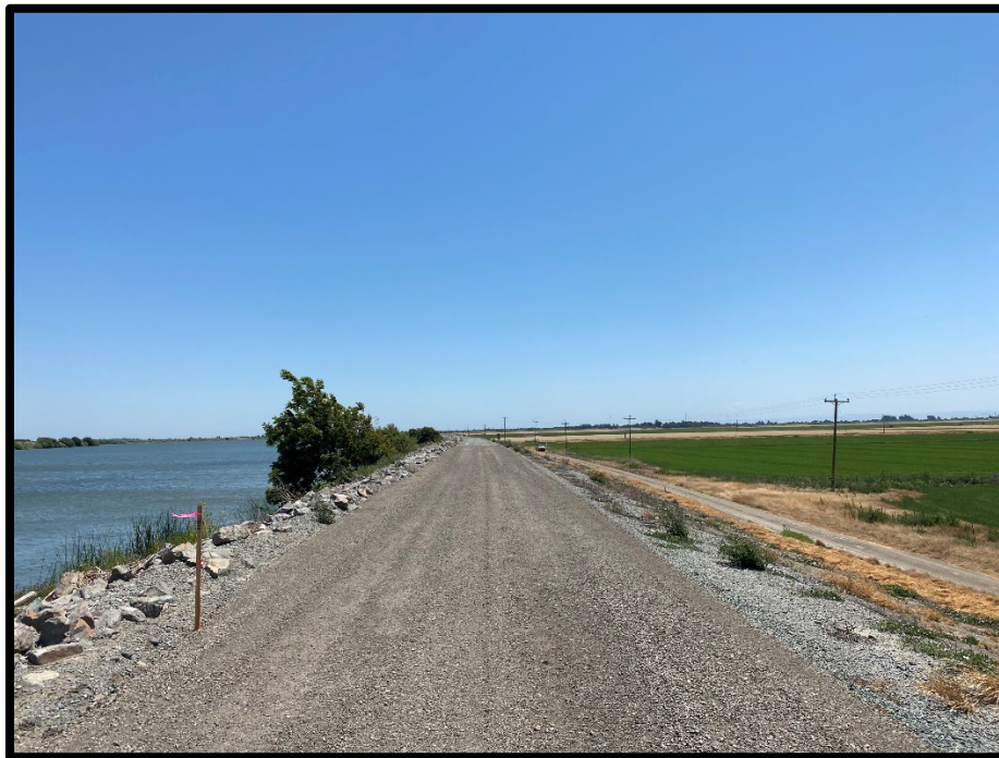
6. As-built gravel repair Site 3 end, Station 191+00
