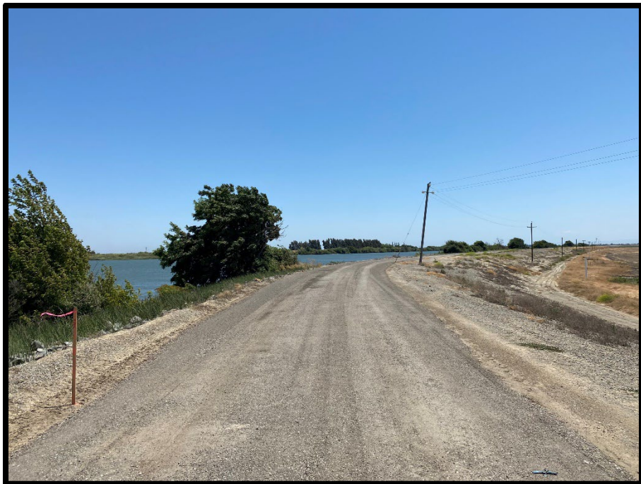
14. As-built gravel repair Site 7 end, Station 254+00
