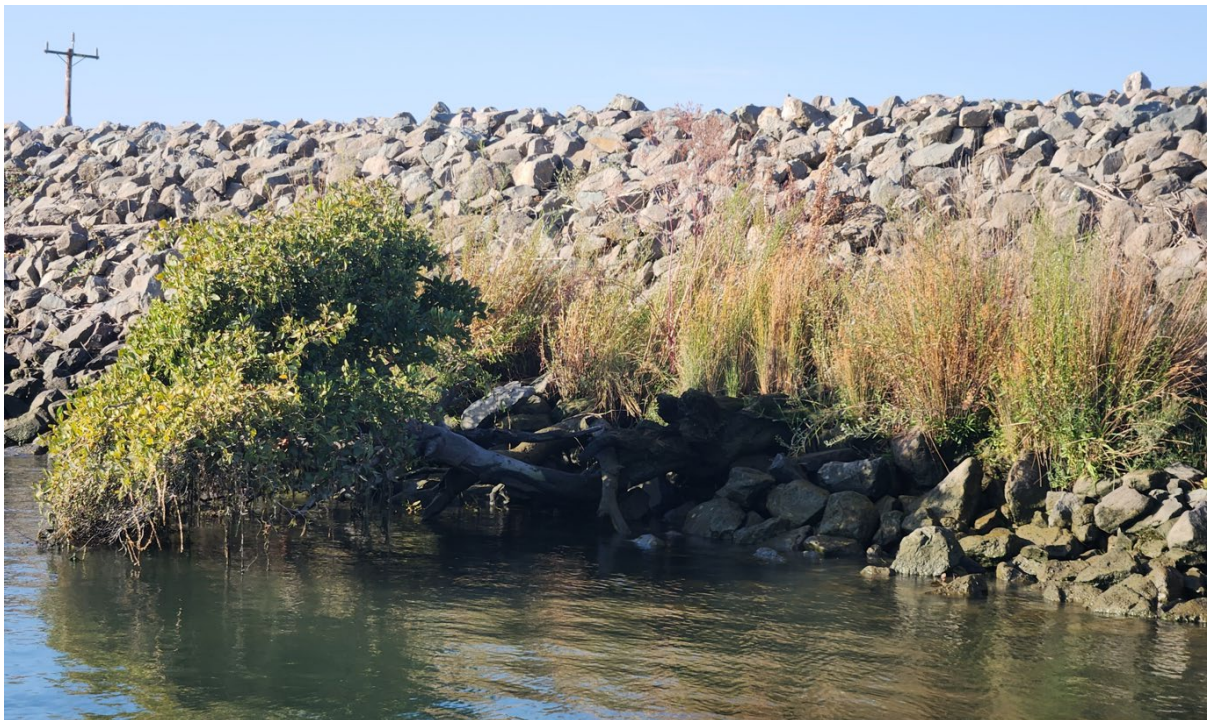
Possible Den Entrance near Station 201+50
