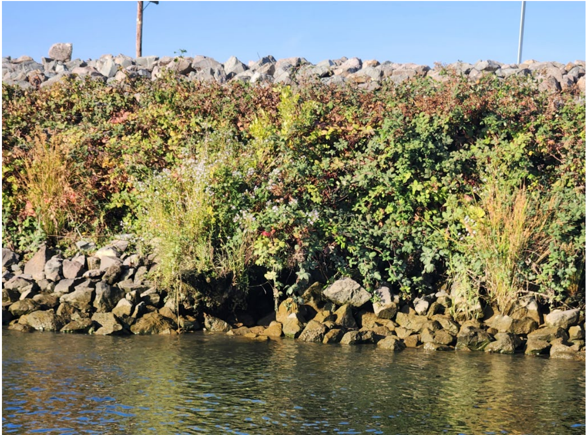
Possible Den Entrance near Station 200+00
