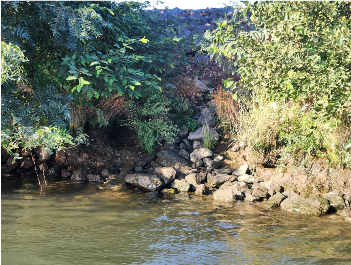
Possible Den Entrance near Station 230+00
