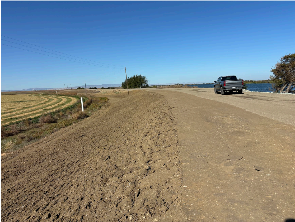
Setback As-Built facing north near station 256+00
