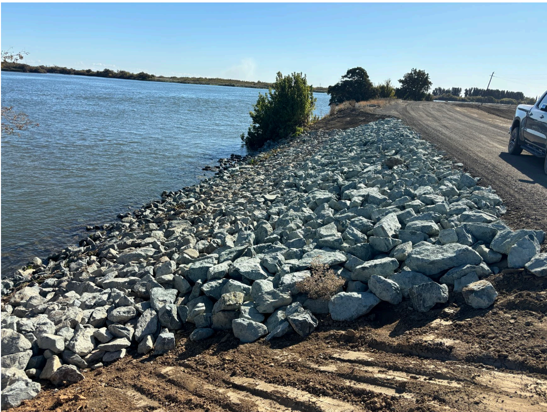
Setback Waterside Facing South near station 256+00
