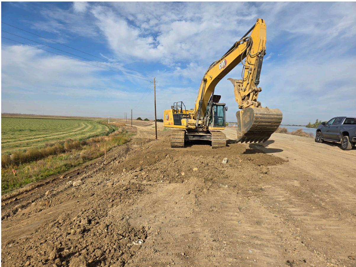
Excavator grading LS shoulder near station 256+00
