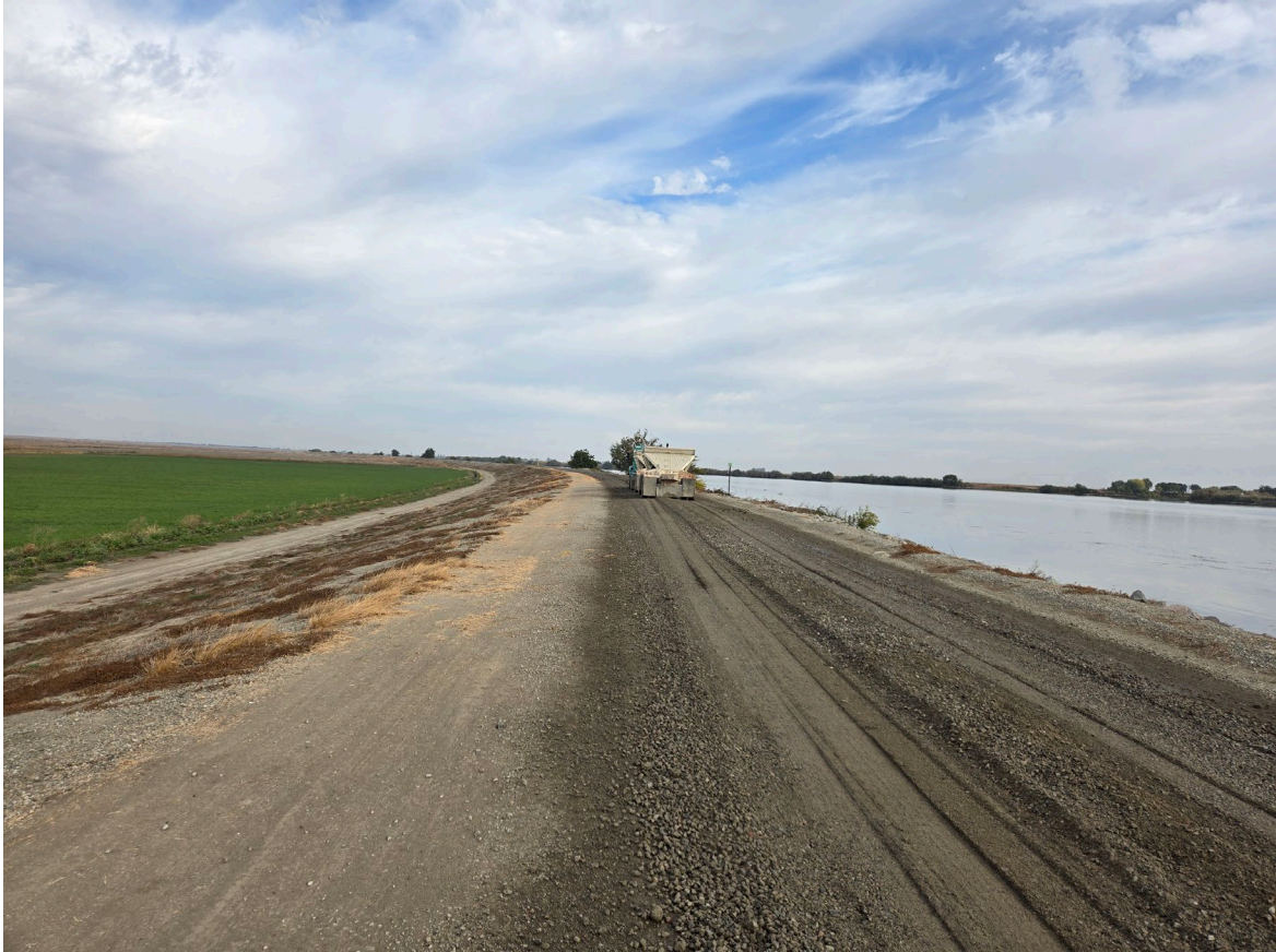
Gravel Truck Dropping Rock on Levee Crown near Station 120+00
