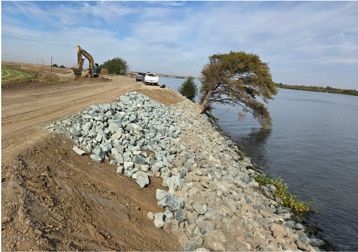
Excavator Preparing LS shoulder; view of WS repair at station 256+00
