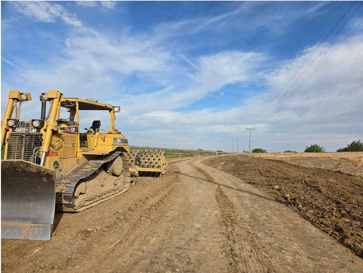
Dozer and Compactor near statio 215+00 site 1 toe berm
