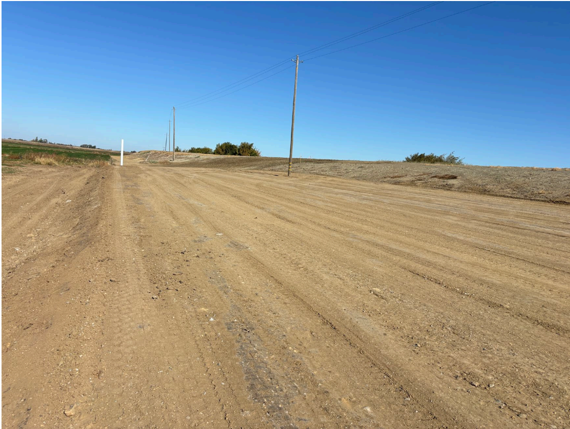
As-Built Toe Berm facing north near 217+00
