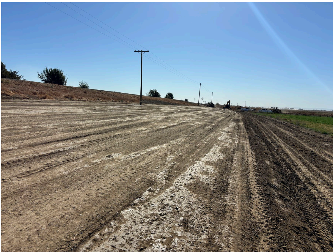
As-Built Toe Berm facing south near 217+00
